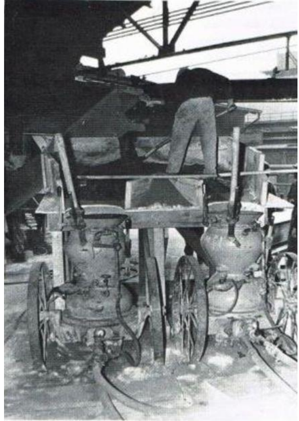
Torcrete Maschine Allentown 1965
